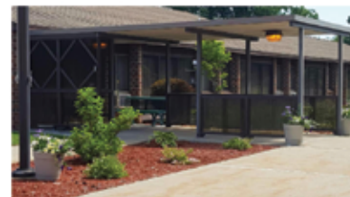
SHAWL I 225 South Hall Street in Whitehall
